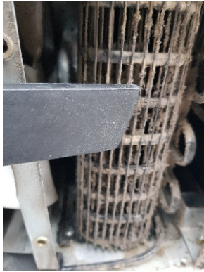
Figure 11: Use vacuum nozzle to remove debris and clean up the area.
