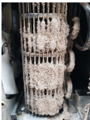
Figure 8: Heavily blocked condenser.
