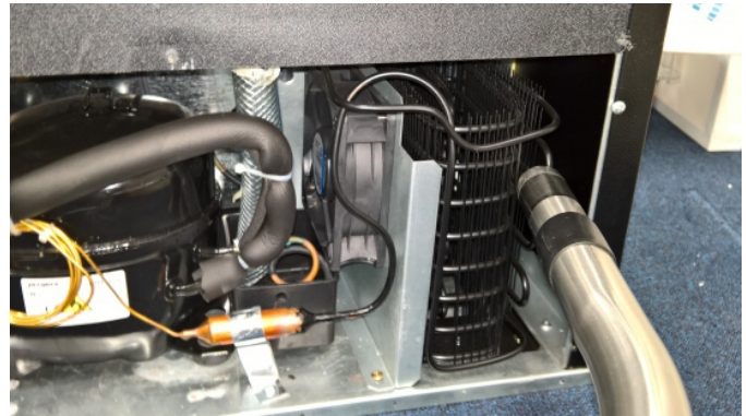
② Use vacuum to remove debris
