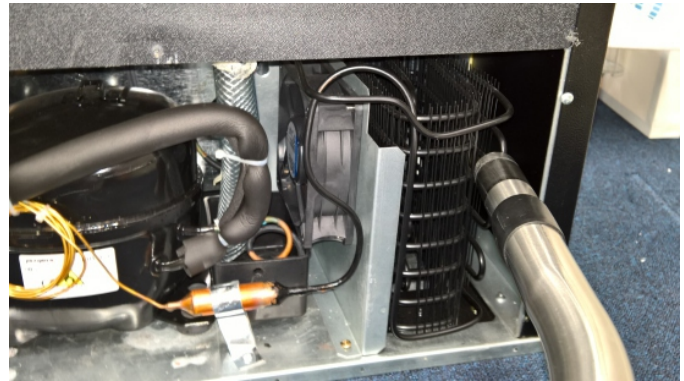
② Use vacuum to remove debris
